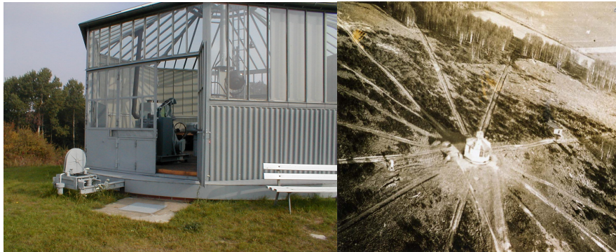
Fig. 6.12 Azimuth pulley of the restored winch house at Lindenberg [23] (left) and historic aerial photo of the winch house showing the forest aisles required for launching [4] (right).
